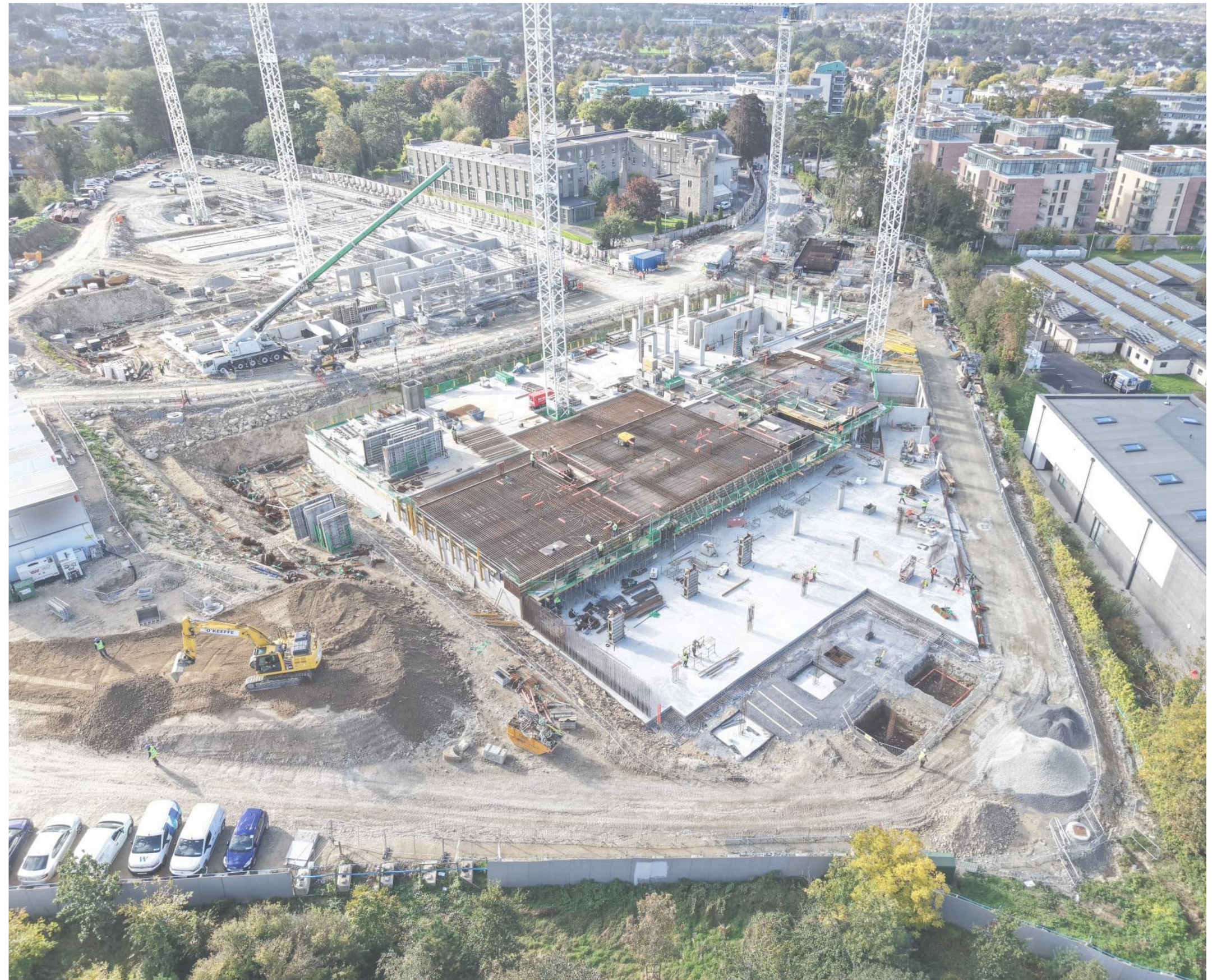
Figure 2 - Aerial view of the site under construction
